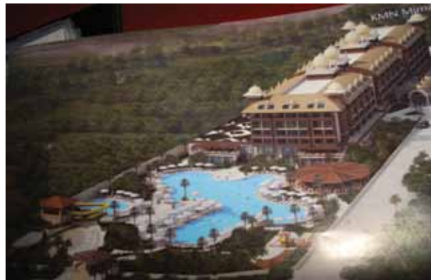
TURKEY Flat Roof and Swimming Pool
