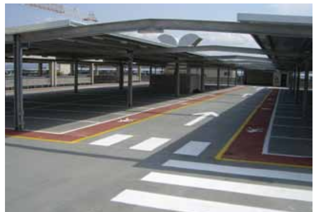
SPAIN Parking Deck, Girona Airport
