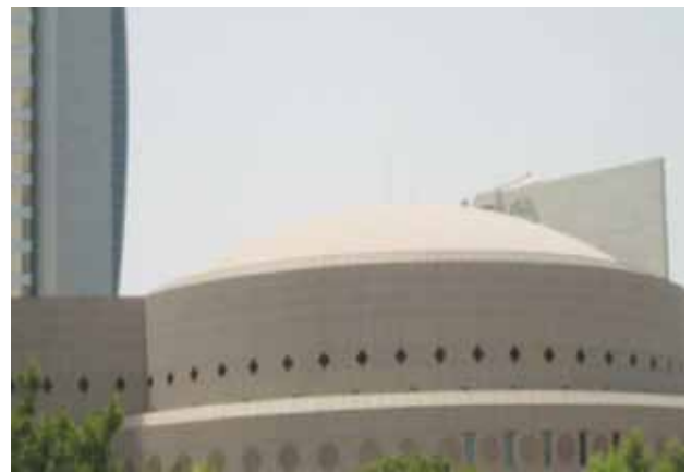
UNITED ARAB EMIRATES-DUBAI Dome Roof
