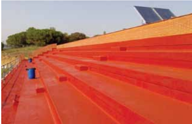
SPAIN Waterproofing of Stadium Tibunes
