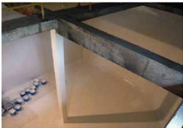
INDONESIA Sewage Treatment
